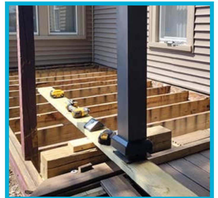
James' deck while its under construction.
