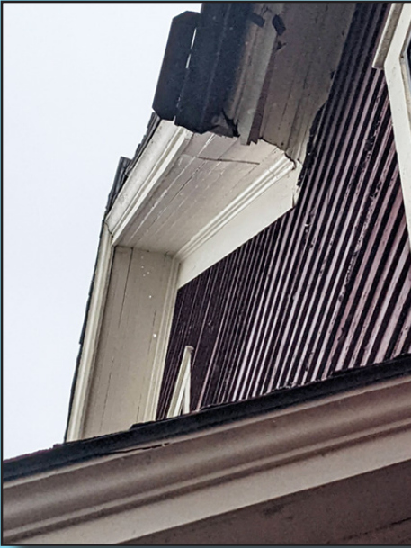
An image showing the previous state of Franklin's roof.
