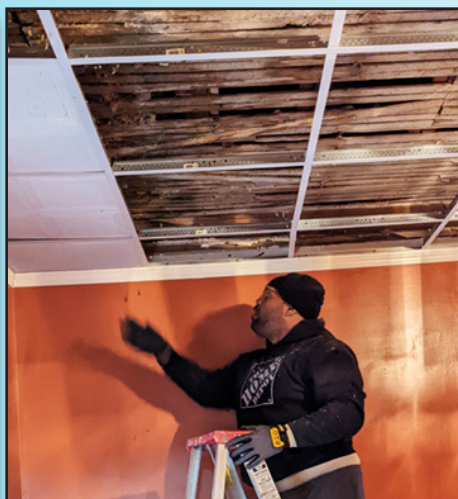
A volunteer removes the water-damaged drop ceiling.
