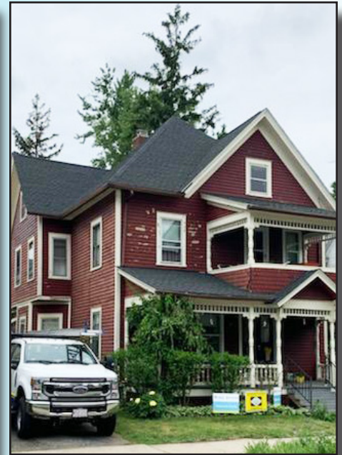
The new roof is done.
