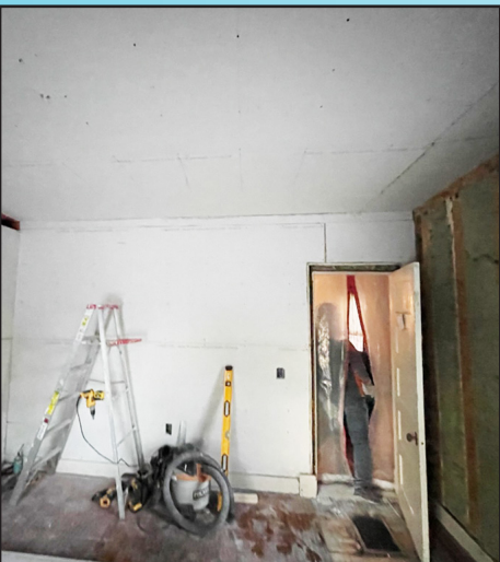
The repair is in process.
