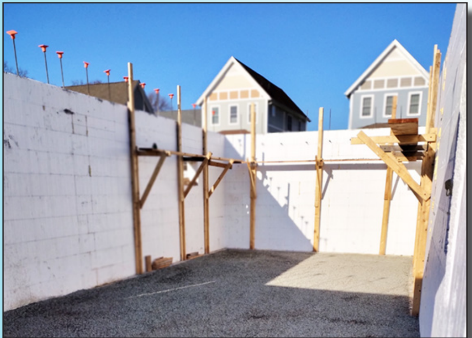
Looking into the basement from the walkout entrance.
