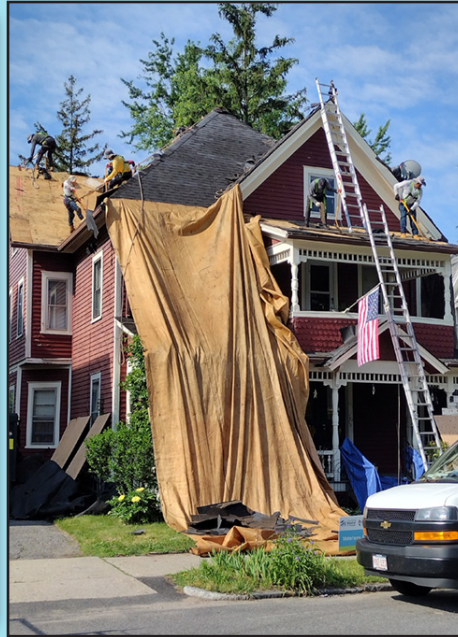
Nextgen roofing takes off the old roof.
