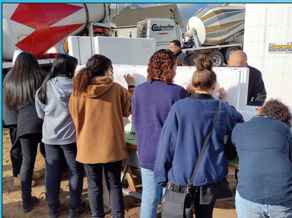
From left: students from Springfield’s Roger L Putnam Vocational Technical Academy autograph foam blocks Nov. 18 at the “Behind the Build” event in Holyoke. On the right, two of the future homeowner’s daughters and son sign foam blocks.
