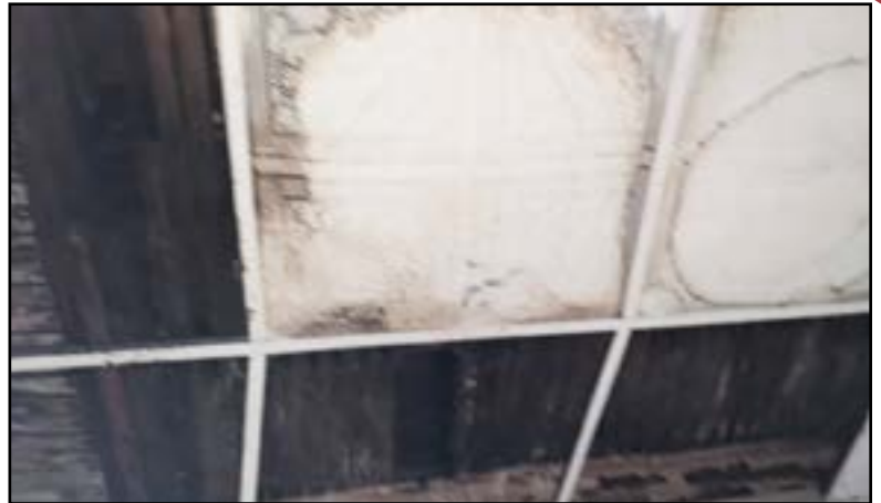
Left: The front of Franklin's Springfield home. Below: Water damage ruined ceiling tiles in a room at Franklin's Springfield home.
