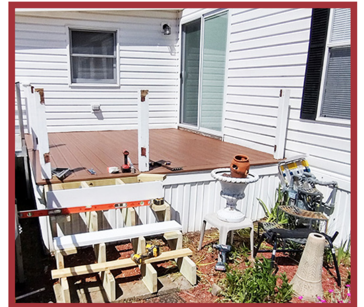
Wayne's new deck while its under construction.
