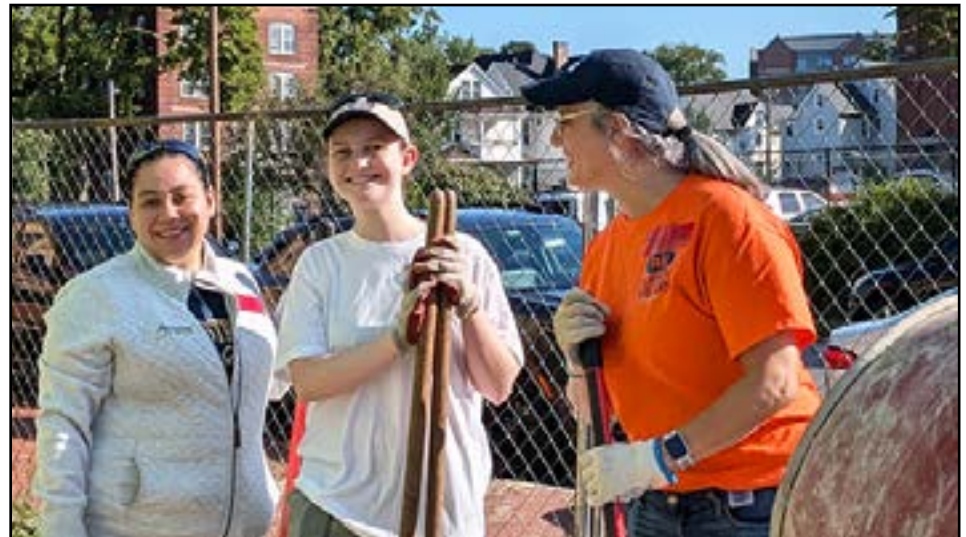
Holyoke's Appleton Corp volunteers take a quick break to smile at the camera. They're working at the Dwight Street, Springfield, build site.
