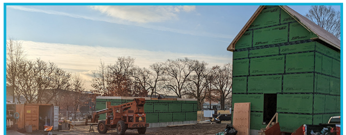
Construction for these Holyoke homes will use CPA funds.
