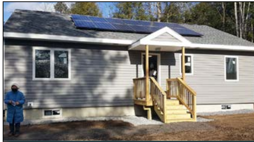
Habitat for Humanity North Central Massachusetts A newly-constructed three-bedroom, two-bathroom all-electric home in Ashburnham.
